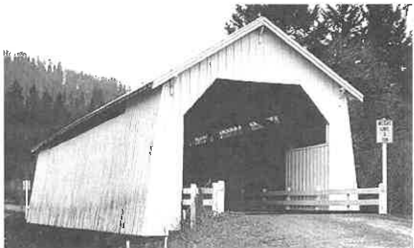
Hayden Bridge, Benton County
